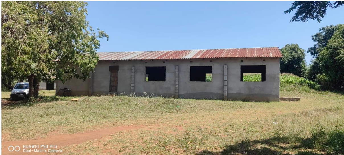
The new business centre block under construction
